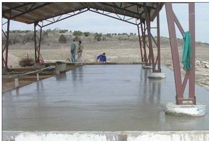
The new floor with mirror-smooth finish
