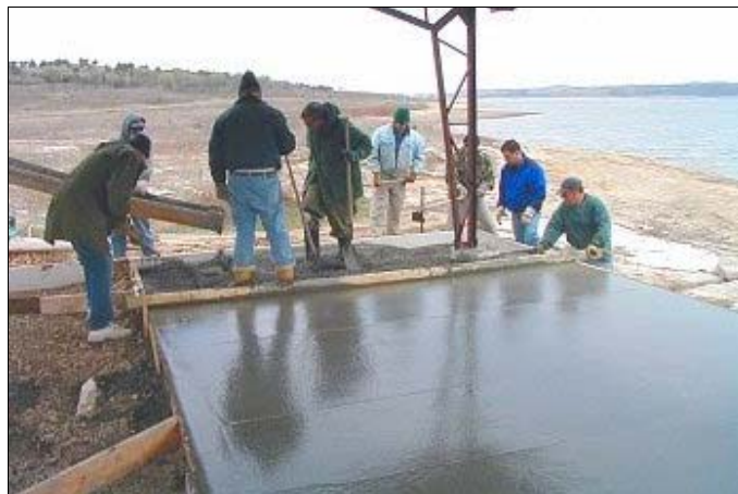
Leveling the cement by "sawing" with a 2 x 4
