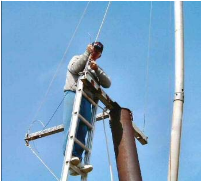
Above: Bob Mullen makes the final adjustment to one of the guy wires
